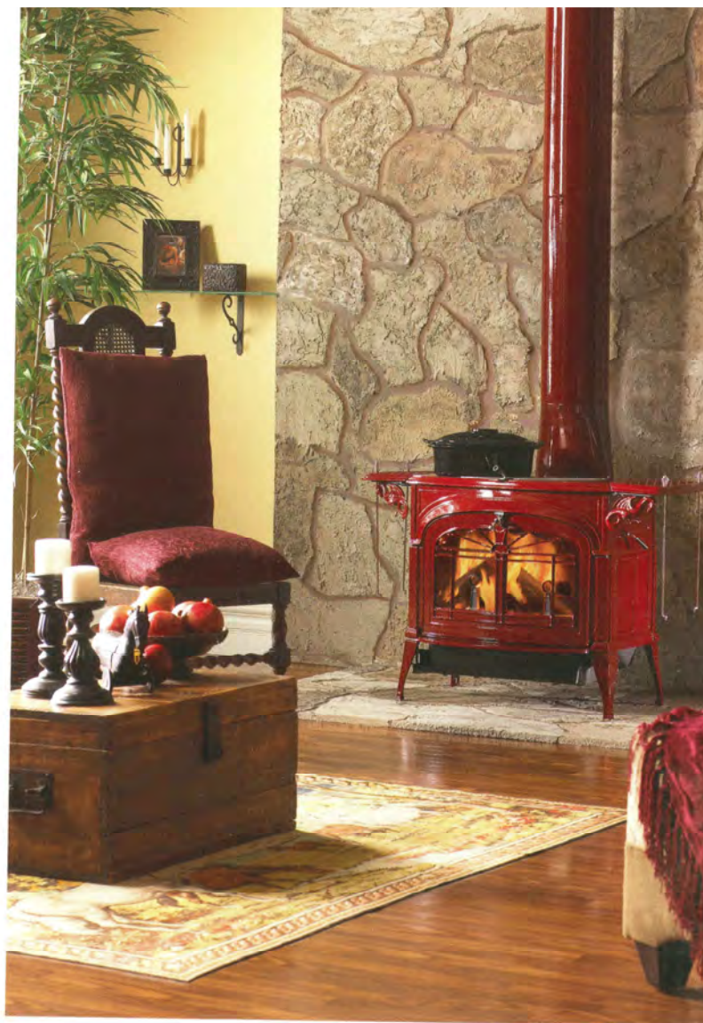
ABOVE: A masonry heat shield and insulated hearth like this faux stone arrangement is a deterrent for fire and also protects the fireplace framing and floor from intense heat.
